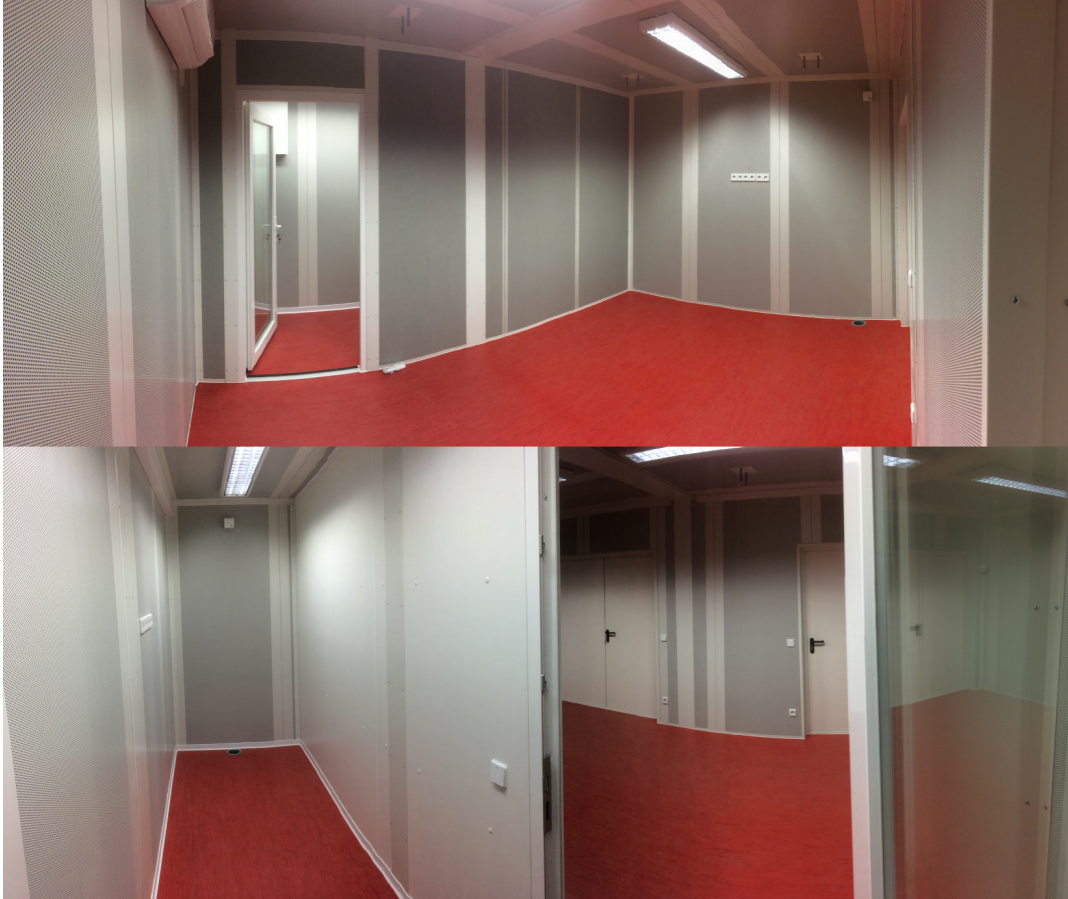
FIGURE 4.4: Photos of the finished interior of the laboratory container. Each of the two rooms has a separate air conditioning and a door prevents air circulation from the main room to the more sensitive laser components. An anti-static floor was laid and baseboards were applied. The walls consist of a 15 cm thick insulation layer and a 5 cm soundproofing layer. Additionally, a hole pattern was applied to the otherwise plain inner walls. The soundproofing reduces the noise by other works in the experimental hall to an inaudible level.
